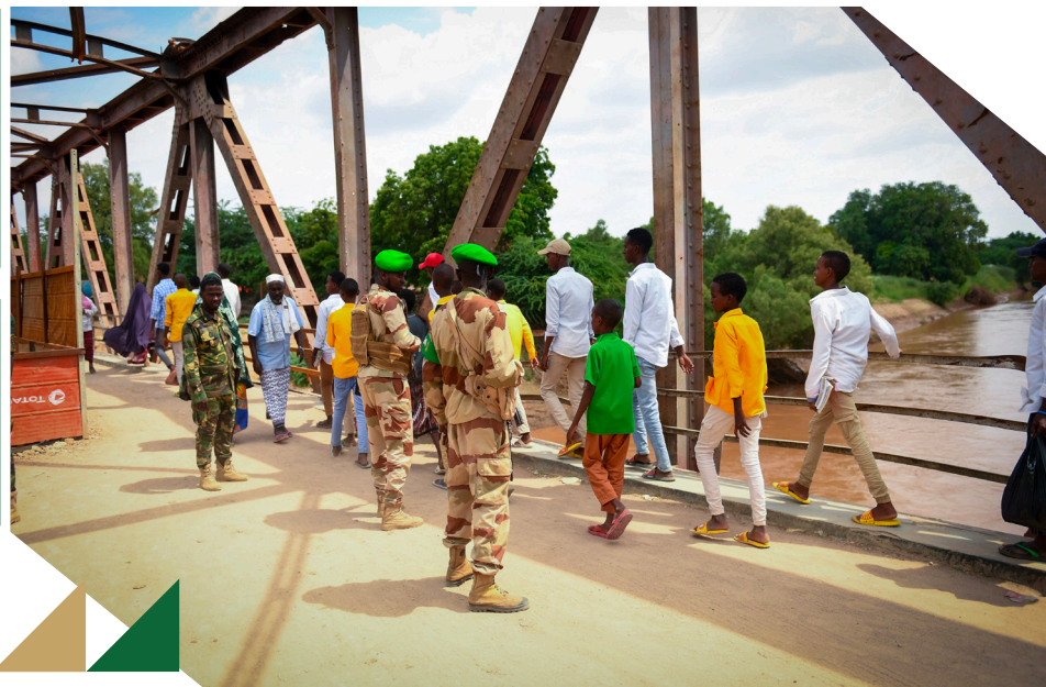
Djiboutian soldiers serving with the African Union Transition Mission in Somalia (ATMIS) at the bridge that connects Bulo Burto district over River Shabelle, in Hirshabelle State. - 27 November, 2022.
