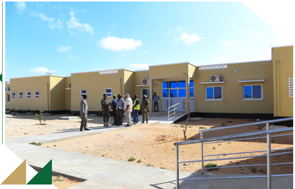
A team from ATMIS touring the newly constructed SNA hospital in Mogadishu. - 26 January, 2023
